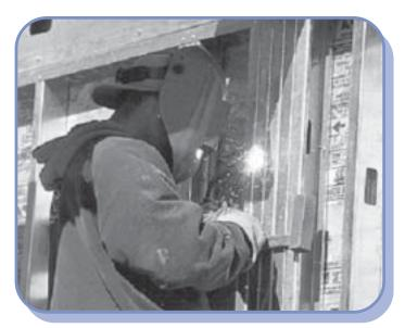
Figure 4.12–Welding of Cold-Formed Steel Framing
