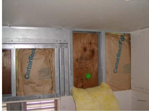
**Figure D.38: S wall – plywood with insulation**
