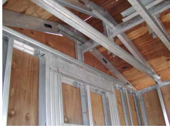
**Figure D.8: Interior wall and roof framing**
