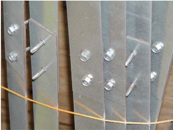
**Figure C.64: Location 3 – connection fasteners**
