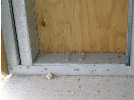
**Figure D.23: SW corner cripple wall base**
