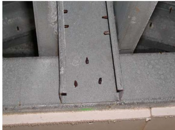
**Figure E.59: Ceiling to king post fasteners**
