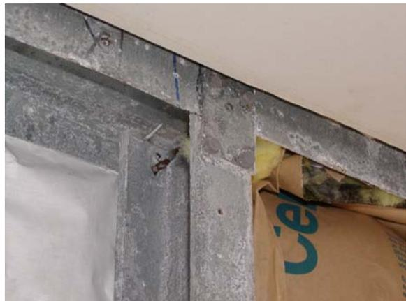
**Figure E.52: N wall – stud to top track connection**
