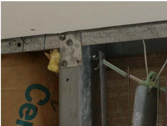
**Figure D.110: Location 2 – top plate connection**
