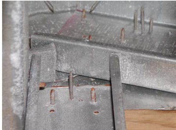
**Figure C.75: Location 2 – Ridge truss connection**
