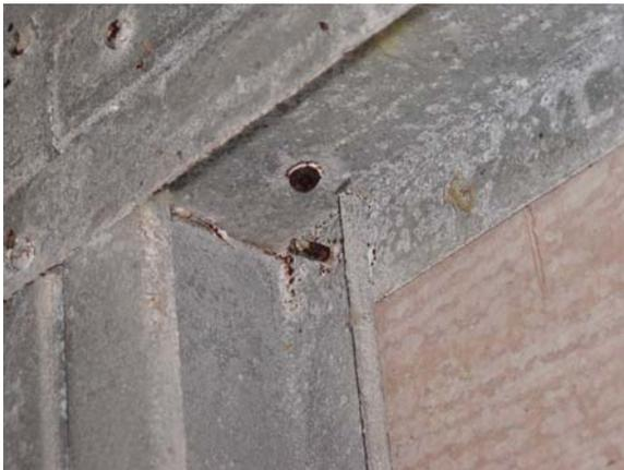
**Figure E.44: W Wall top track connection**
