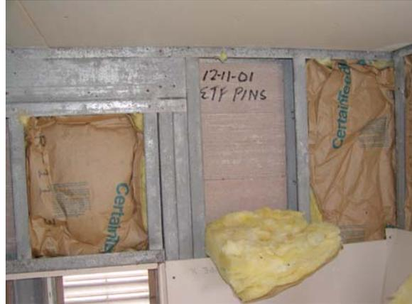
**Figure E.41: W wall – Lap siding with insulation**
