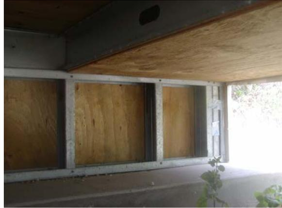
**Figure D.53: NW corner cripple wall**
