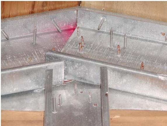
**Figure A.34: Ridge connection fasteners**
