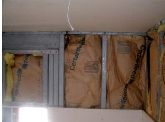
**Figure E.91: E wall – Plywood with insulation**
