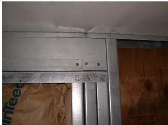
**Figure D.40: S wall – West header connection**
