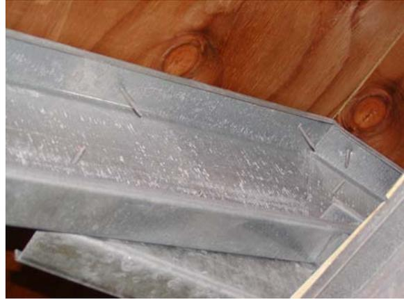
**Figure D.48: Roof truss ridge connection**
