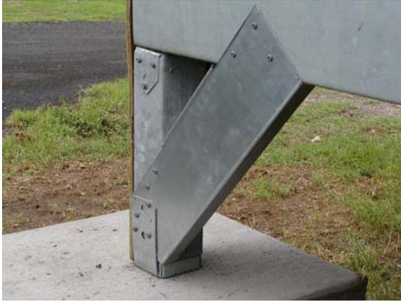
**Figure D.7: NE post and brace**
