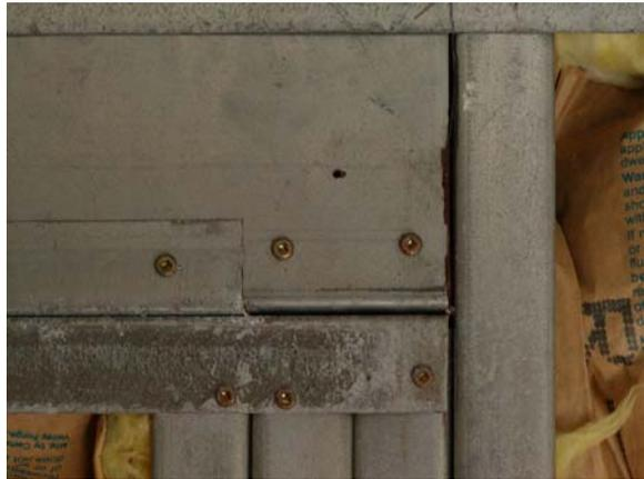
**Figure D.117: Location 3 – Header connection**
