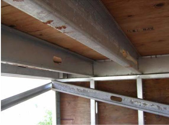
**Figure B.20: Joists on Cripple Wall – NE corner**
