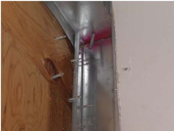
**Figure C.32: South Wall – West corner fasteners**
