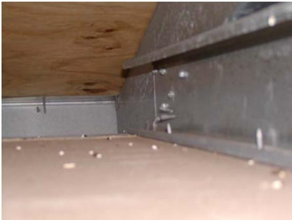
**Figure D.51: Roof truss eave connection**
