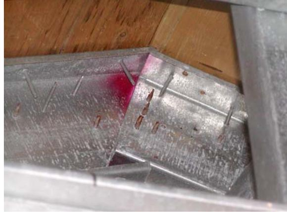
**Figure B.32: Ridge connection fasteners**
