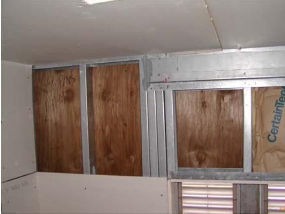
**Figure D.37: S wall – plywood w/o vapor barrier**
