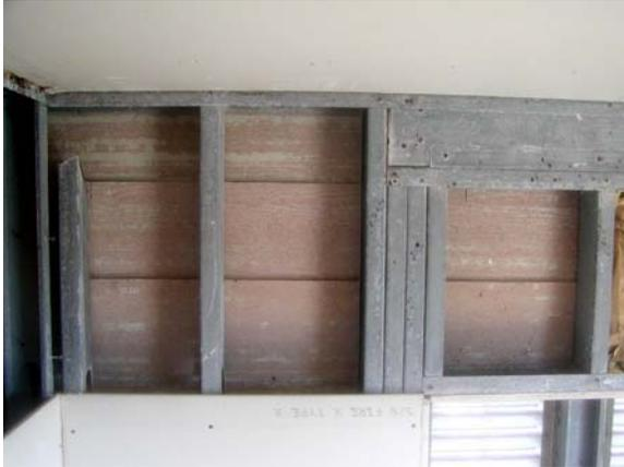
**Figure E.84: W wall – Lap siding w/o vapor barrier**
