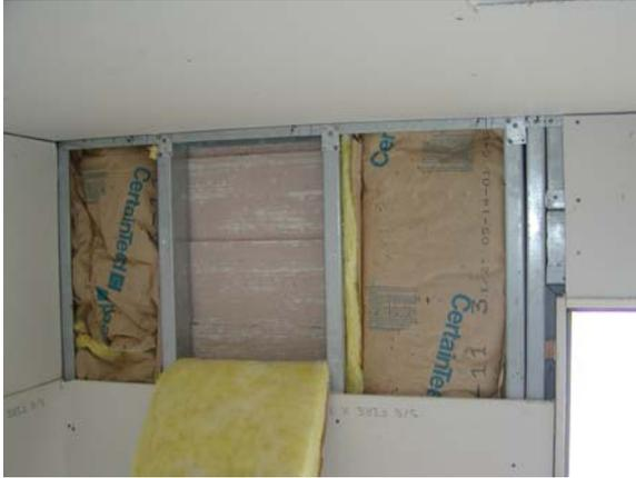
**Figure D.33: E wall – Lap siding w/o vapor barrier**
