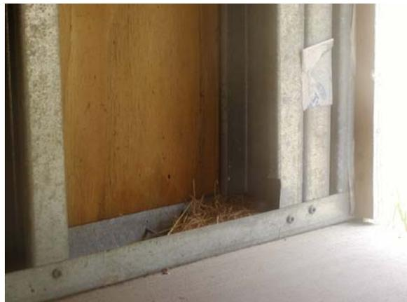
**Figure D.55: NW Cripple Wall base connection**
