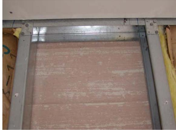
**Figure D.34: E wall – Studs and top track**
