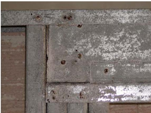
**Figure E.42: W wall header connection**
