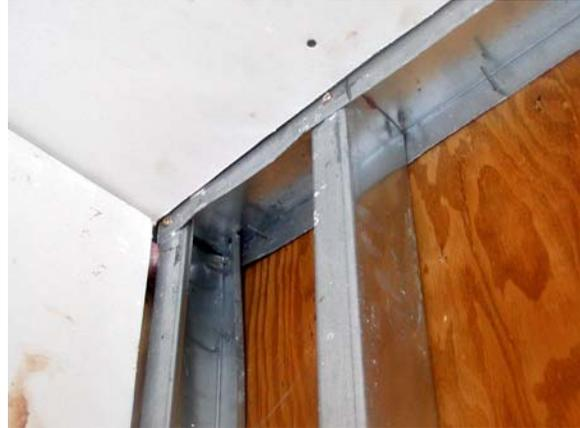
**Figure B.27: East Wall – Top Track detail**
