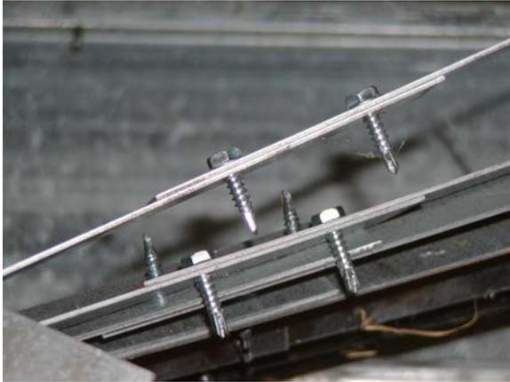
**Figure D.98: Connection fasteners – covered crawl**
