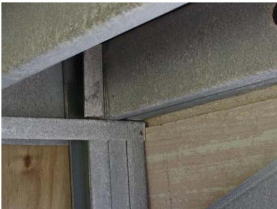
**Figure E.15: Double Joist at SW corner**
