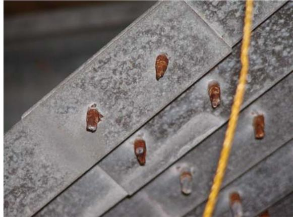
**Figure D.101: 7 Month exterior fasteners**
