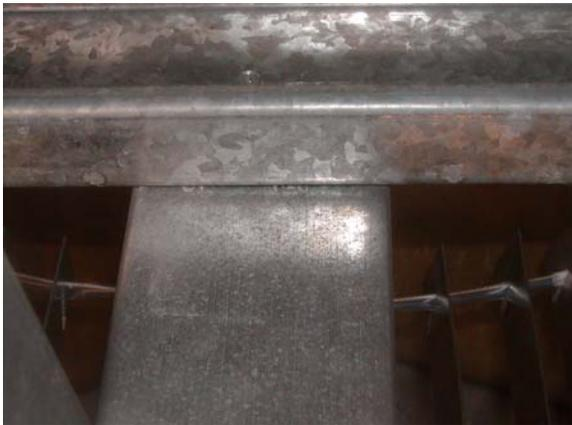
**Figure C.41: Post to cross brace connection**
