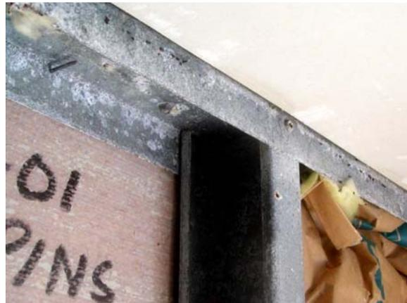
**Figure E.89: W wall – top track detail**
