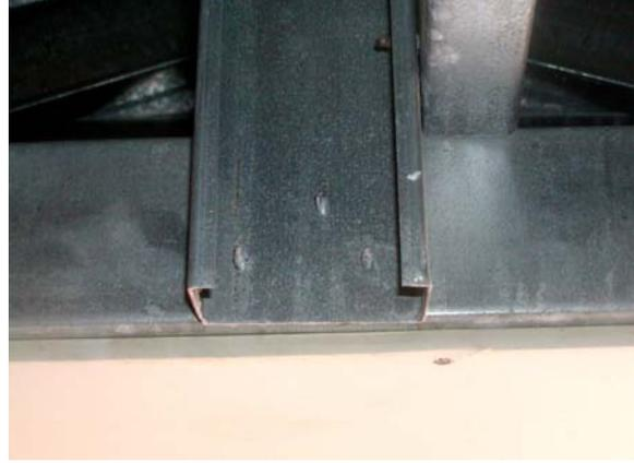
**Figure C.40: Post to ceiling joist connection**
