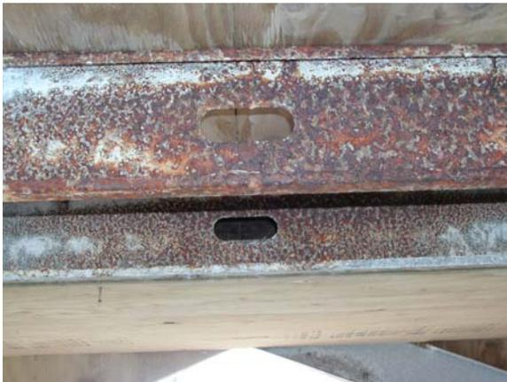
**Figure E.36: Exposed joist detail at midspan**
