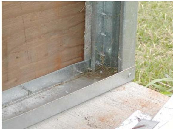
**Figure A.45: Cripple Wall – SE corner bottom**
