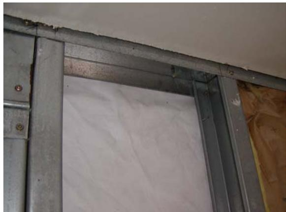
**Figure D.45: N wall – Top track connections**
