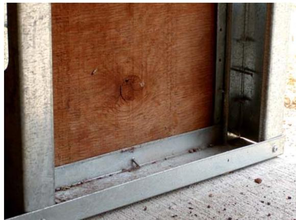
**Figure C.10: Cripple wall base - SE**
