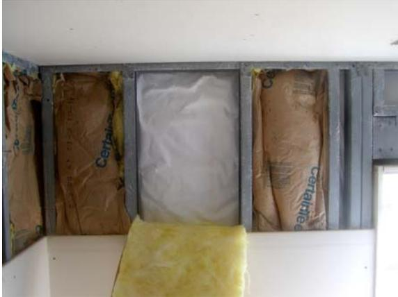
**Figure E.96: N wall – vapor barrier & insulation**
