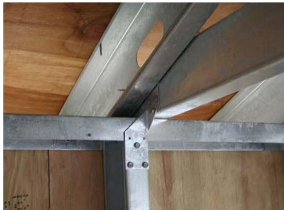
**Figure D.10: Roof truss eave connection**
