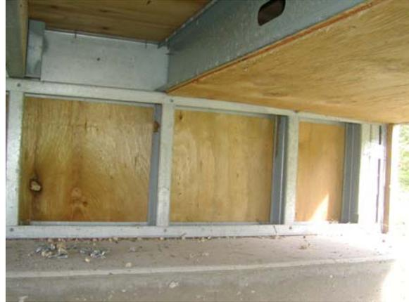
**Figure D.79: Cripple Wall – NW corner**
