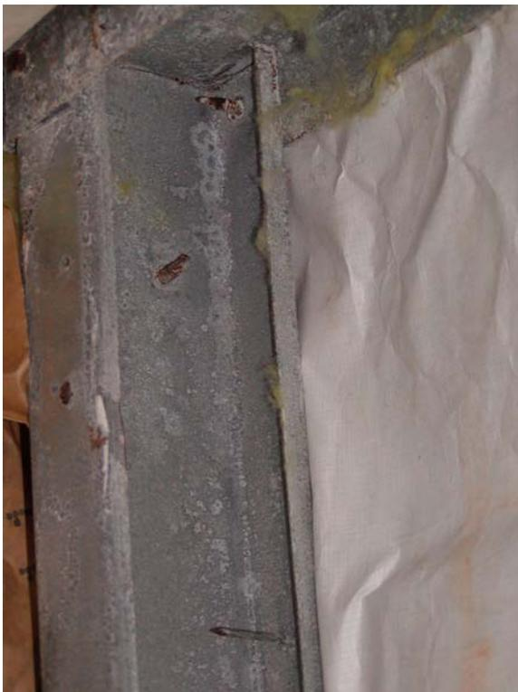
**Figure E.53: N wall – stud and siding fasteners**
