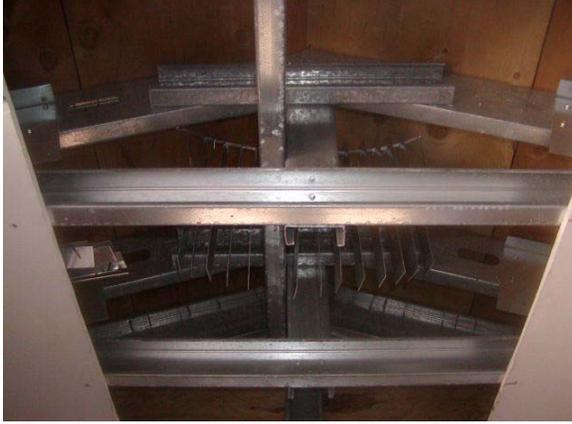
**Figure C.39: Attic framing with test connections**
