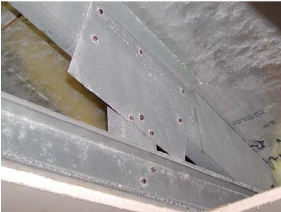
**Figure E.58: Eave connection fasteners**
