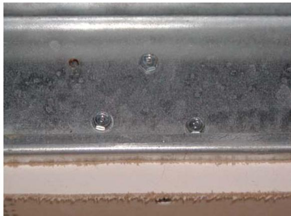
**Figure D.50: Roof truss fasteners**
