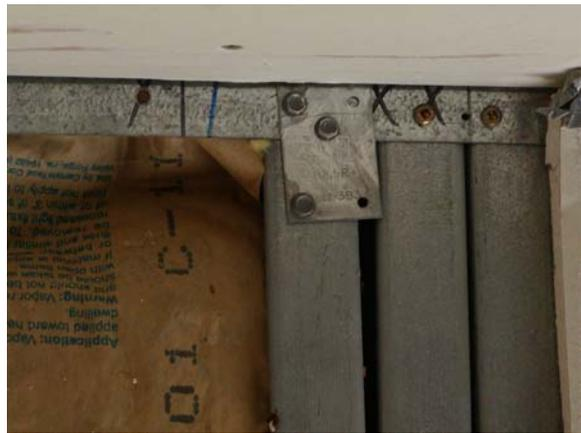
**Figure D.111: Location 2 – top plate connection**
