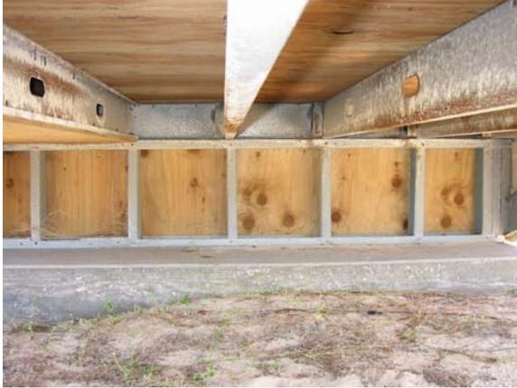
**Figure E.19: Exposed Joists and Cripple Wall**
