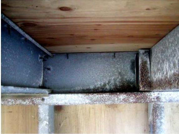
**Figure E.72: Joists bearing on cripple wall**
