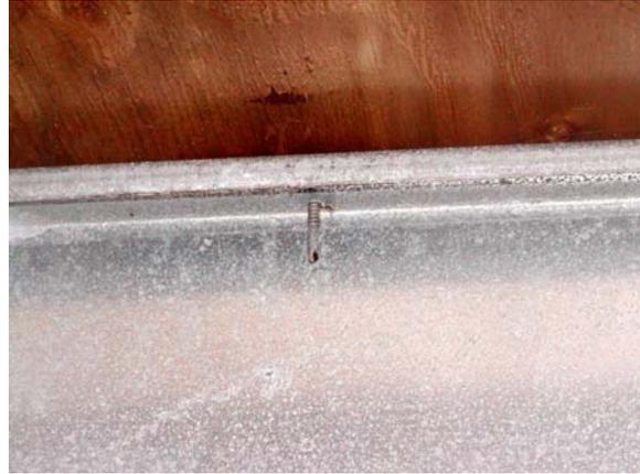
**Figure E.79: Covered joist and fastener**
