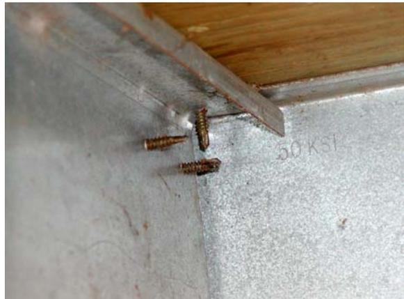
**Figure C.22: Joist to track fasteners**
