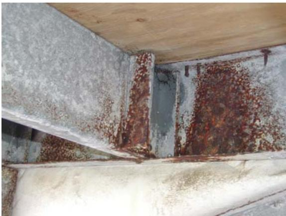
**Figure E.140: Joist stiffener at South end**
