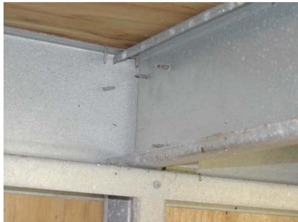
**Figure D.81: Cripple Wall Top – Joist connection**
