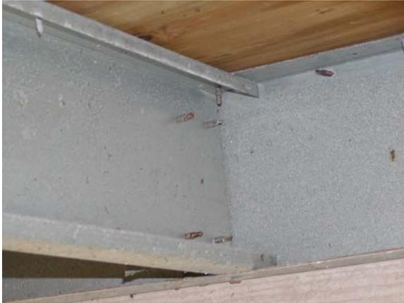
**Figure D.92: Joist end connection – open crawl**
