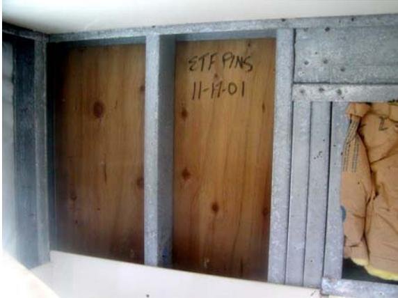
**Figure E.90: E wall – Plywood w/o vapor barrier**
