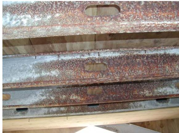
**Figure E.31: Exposed Floor Joists – Midspan - E**
