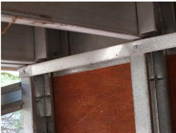
**Figure C.7: Exposed joists on cripple wall - NE**
