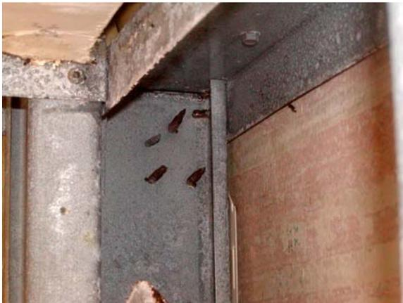
**Figure E.88: W wall – S corner stud fasteners**
