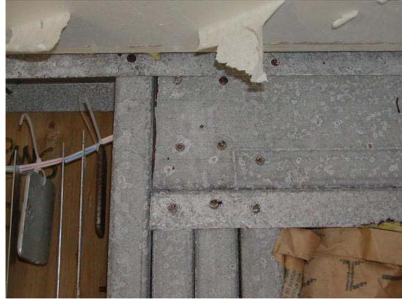
**Figure E.149: E wall - Header connection**
