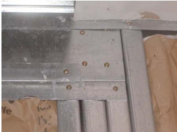
**Figure C.36: North Wall – Header connection E**
