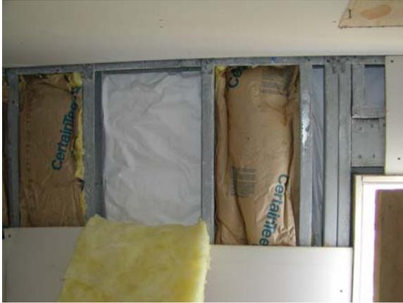
**Figure E.50: N wall – vapor barrier & insulation**
