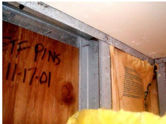
**Figure E.95: E wall – top track fasteners**
