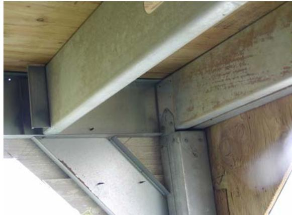
**Figure D.22: Joist and double joist over post**
