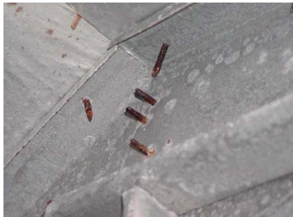
**Figure E.57: Ridge connection fasteners**
