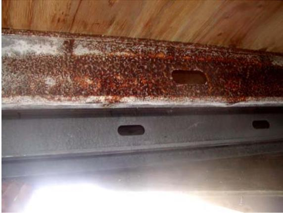
**Figure E.78: Exposed and covered floor joists**
