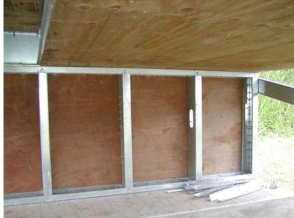
**Figure A.41: Cripple Wall – SE corner**
