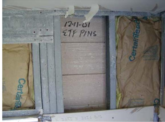
**Figure E.143: W wall- Lap siding with insulation**
