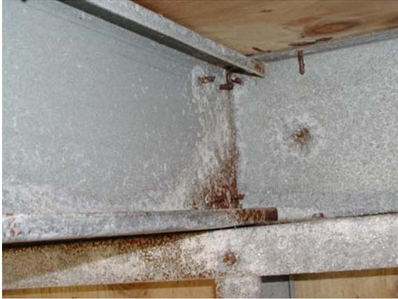
**Figure E.32: Joist connection at cripple wall**
