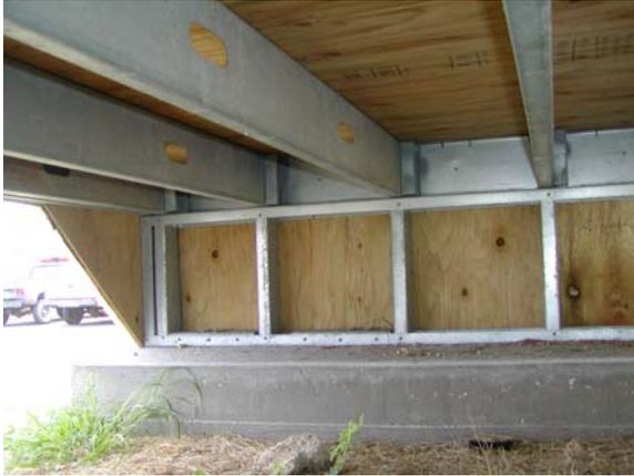
**Figure D.27: SW corner exposed joists**
