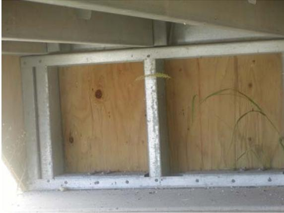
**Figure D.52: SW corner cripple wall**
