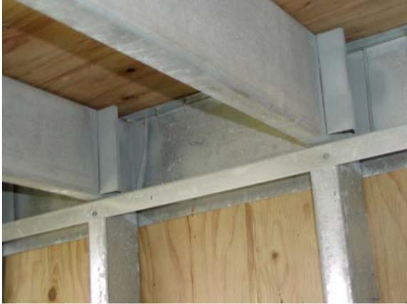
**Figure D.19: Joist ends bearing on cripple wall**
