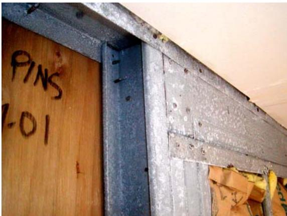
**Figure E.92: E wall – Header and stud fasteners**
