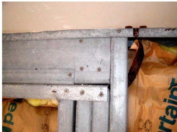
**Figure E.93: E wall – Header connection**
