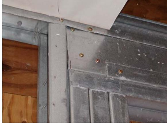
**Figure A.28: North wall – Header west connection**
