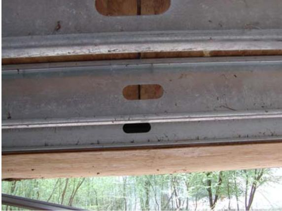
**Figure C.17: Exposed and covered floor joists**
