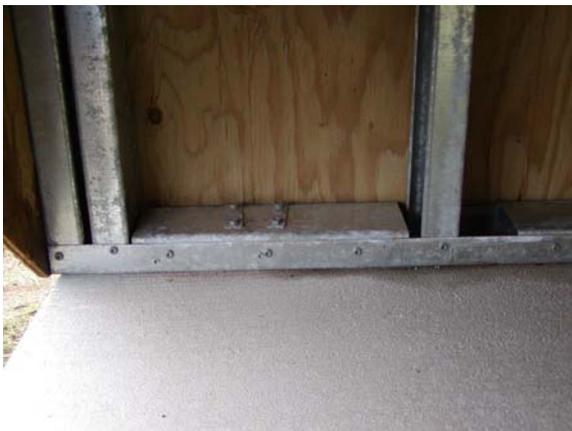
**Figure D.3: SW cripple wall tie-down**
