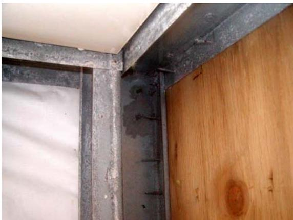
**Figure E.94: E wall – N corner stud fasteners**
