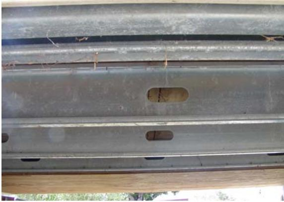
**Figure A.15: Exposed floor joists**
