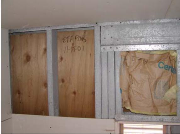
**Figure E.46: E wall – Plywood w/o vapor barrier**
