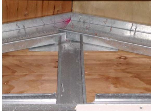
**Figure A.31: End Truss**
