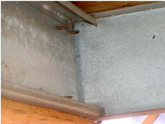
**Figure C.21: Joist connection fasteners**
