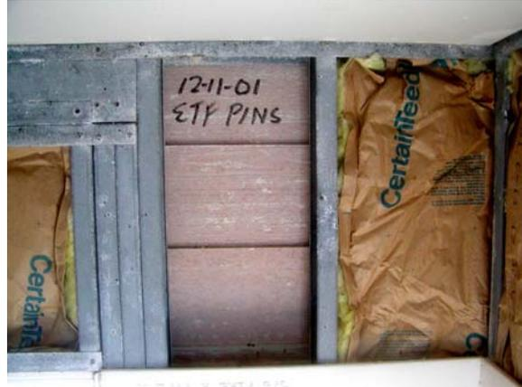
**Figure E.85: W Wall – Lap siding with insulation**
