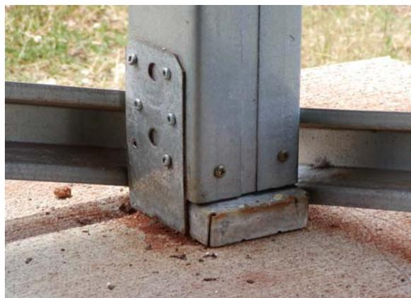
**Figure B.18: NW Post Base – Interior view**
