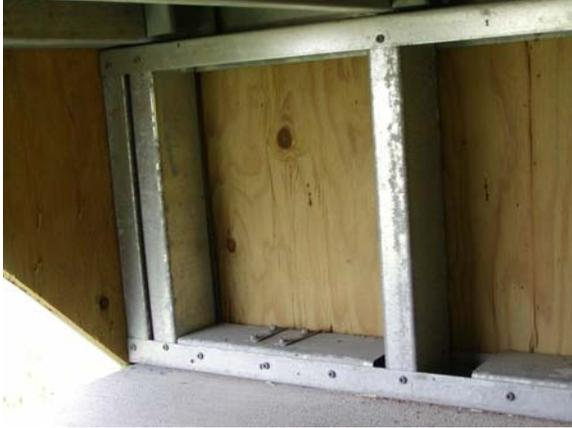
**Figure D.13: SW end of cripple wall**
