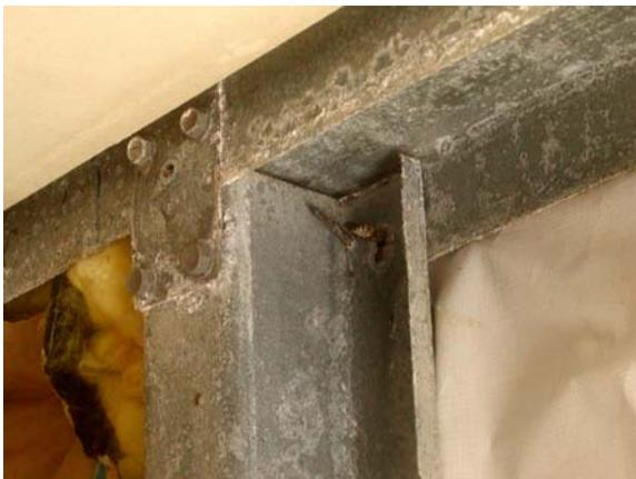
**Figure E.98: N wall – top track connection**
