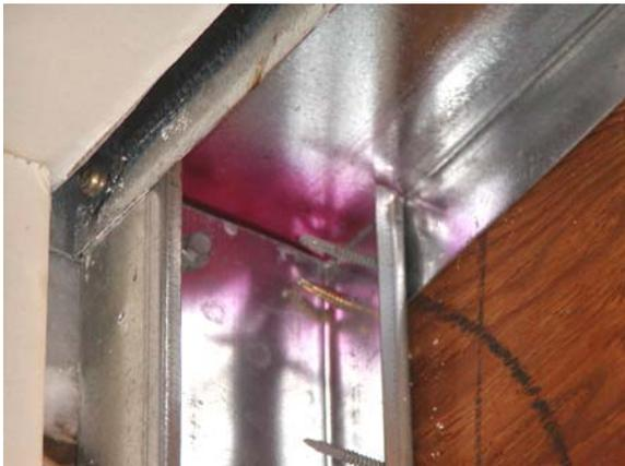
**Figure A.25: East Wall – Top Track Connection**
