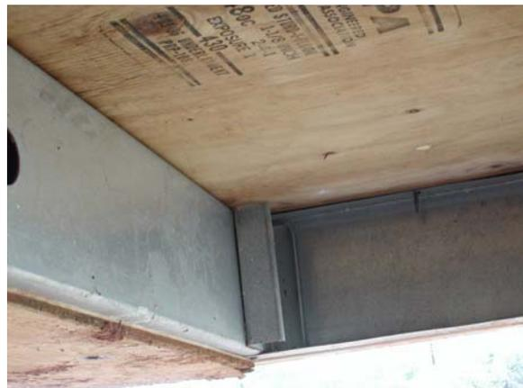
**Figure B.25: Joist stiffener at West connection**
