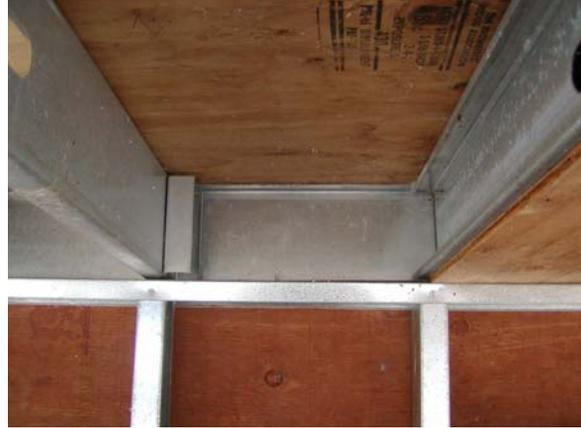
**Figure C.18: Joist connection over cripple wall**
