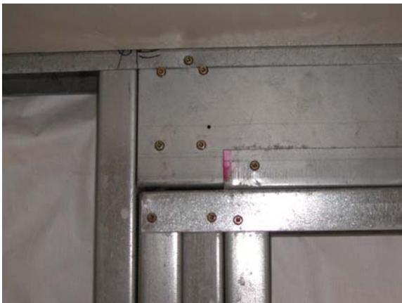
**Figure D.44: N wall – Header connection**
