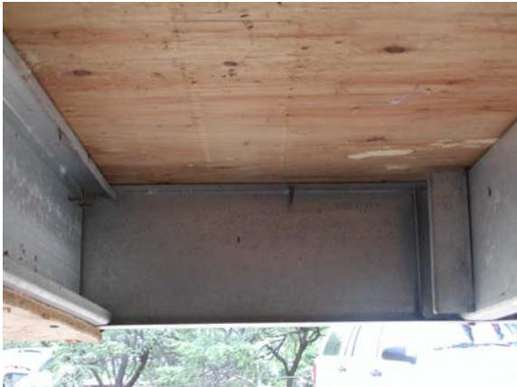
**Figure C.19: Joist connection at South elevation**
