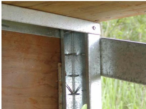
**Figure A.43: Cripple Wall – SE corner top**
