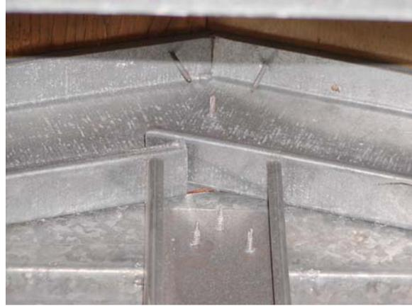
**Figure A.64: Location 2 – Truss top connection**
