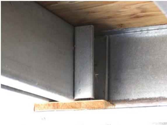
**Figure A.19: Double edge joist with stiffener**
