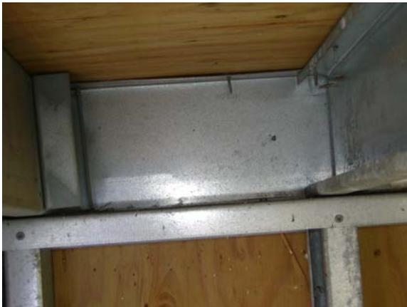
**Figure D.31: Joist stiffener over cripple wall**
