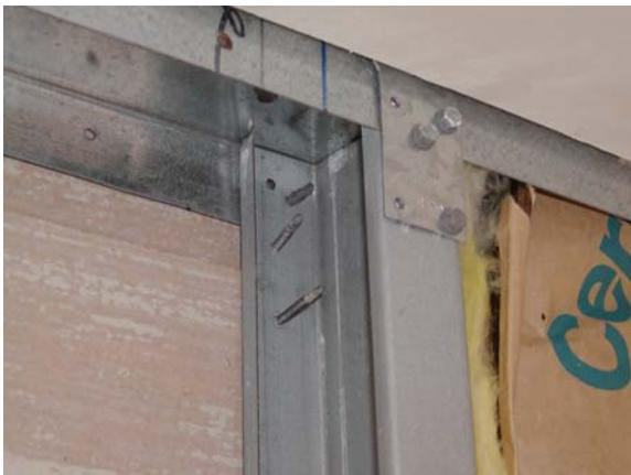
**Figure D.35: E wall – Stud to top track connection**
