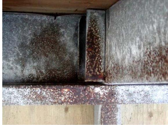
**Figure E.73: Joist stiffener over cripple wall stud**
