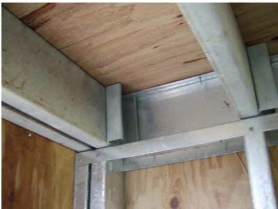
**Figure D.5: Joist stiffeners on cripple wall**
