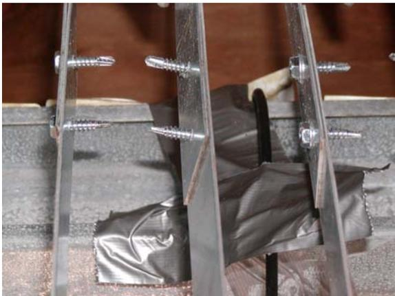
**Figure D.122: Location 4 – connection fasteners**
