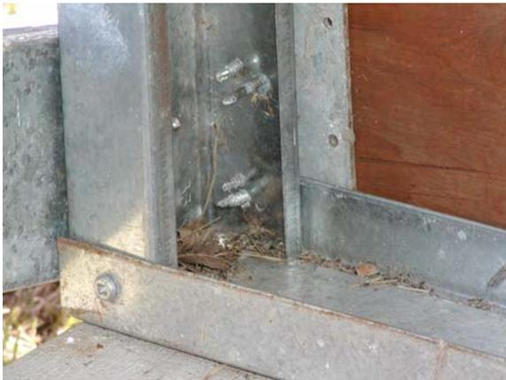
**Figure A.9: Cripple wall base connection – NE end**
