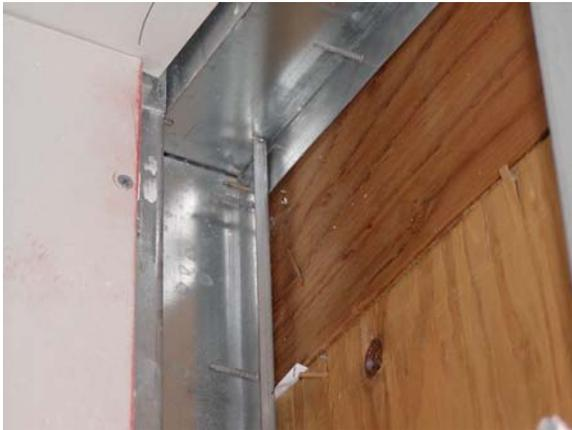
**Figure A.29: North Wall – Top track connection**
