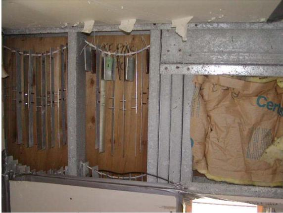
**Figure E.148: E wall – Plywood w/o barrier**
