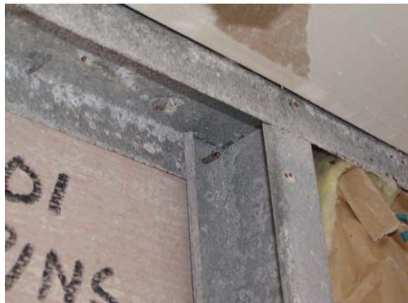
**Figure E.147: W wall top track connection**
