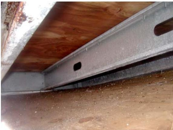
**Figure E.80: Covered Floor Joist – North end**
