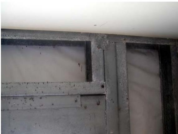
**Figure E.100: N wall – Header and stud connection**
