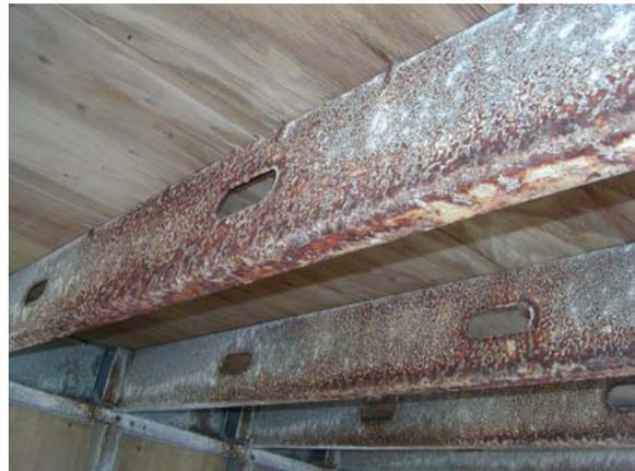
**Figure E.37: Exposed joist soffit at midspan**
