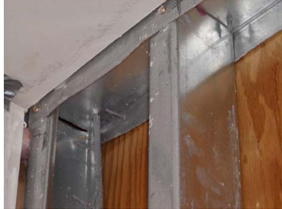
**Figure B.60: Location 1 – Top track connections**
