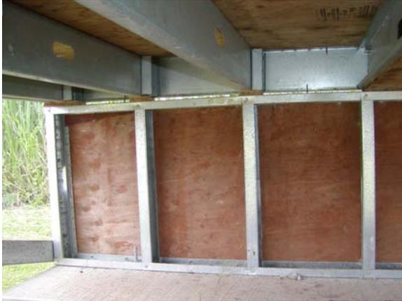
**Figure A.40: Cripple Wall – NE corner**
