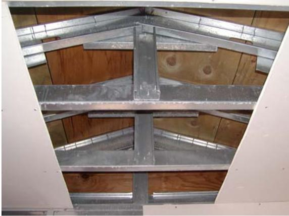
**Figure A.30: Roof Trusses**
