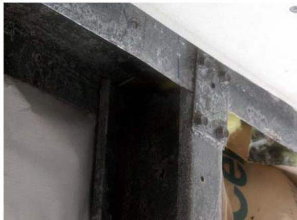
**Figure E.99: N wall – Truss tie-down connection**
