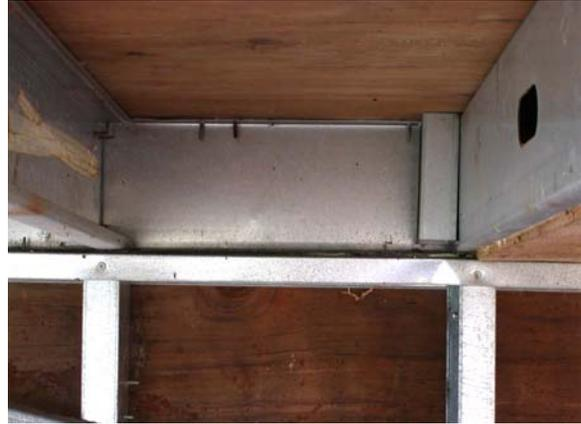
**Figure B.21: Joists on cripple wall – East end**
