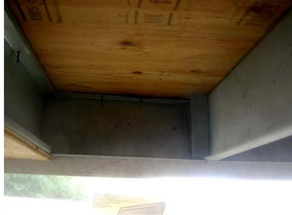
**Figure D.59: Floor joist end connections**
