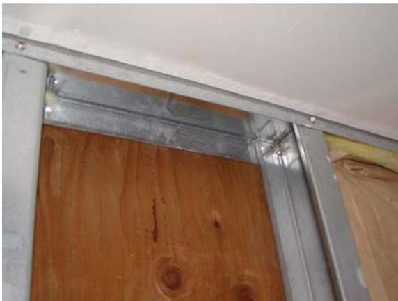
**Figure D.41: S wall – Stud to top track connection**
