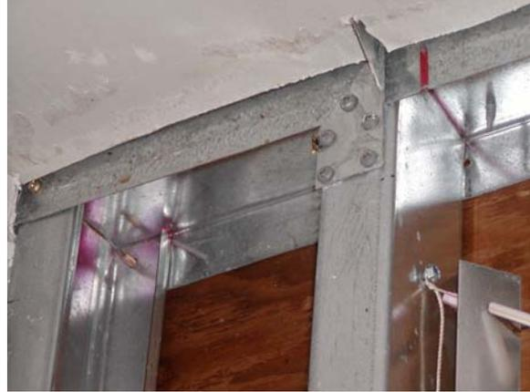
**Figure C.69: Location 1 – Top track connections**
