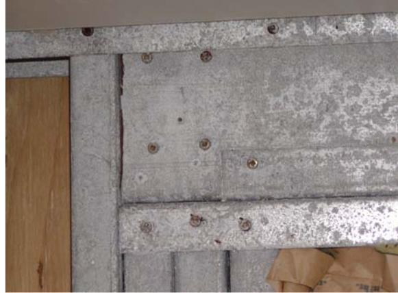
**Figure E.47: E wall – Header connection**
