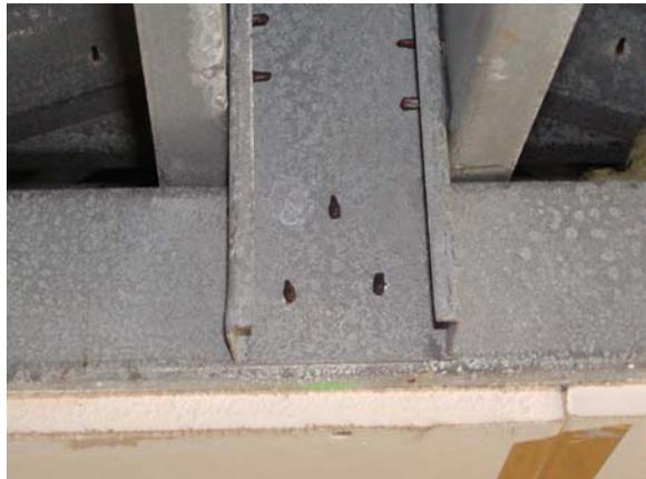
**Figure E.157: Ceiling to king post fasteners**
