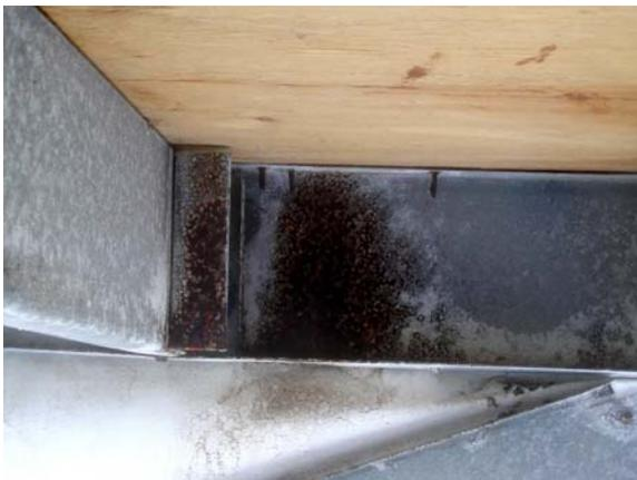
**Figure E.74: Joist stiffener at North end**
