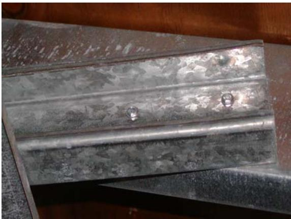
**Figure D.49: Roof truss connection**
