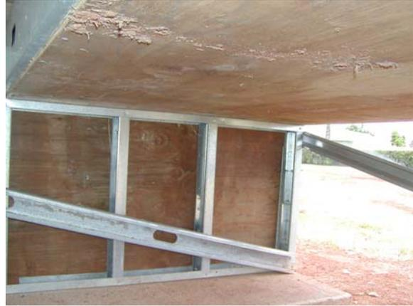
**Figure B.6: Cripple Wall – SE end**
