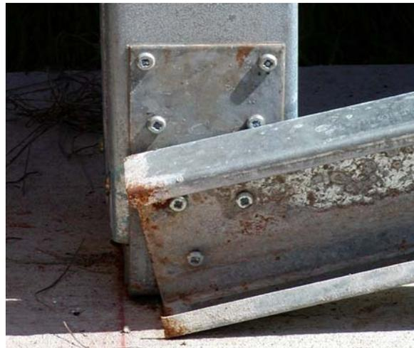
**Figure A.14: SW Post base connection**
