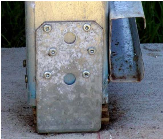
**Figure A.13: NW Post base connection**
