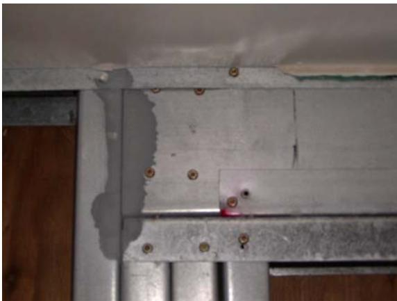
**Figure D.39: S wall – East header connection**
