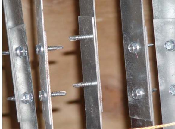
**Figure B.64: Location 2 – connection fasteners**
