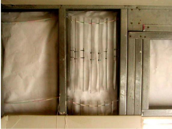
**Figure D.66: Location 3 – wall with vapor barrier**
