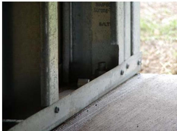
**Figure D.4: NW cripple wall tie-down**
