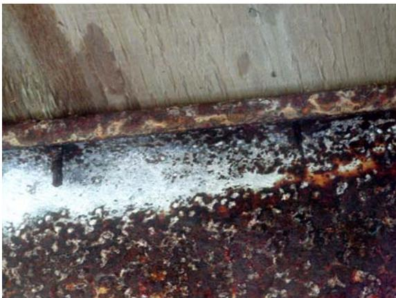
**Figure E.70: Exposed Joists – Close-up of fastener**
