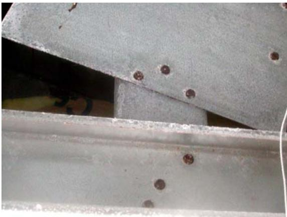
**Figure E.105: Eave connection fastener heads**
