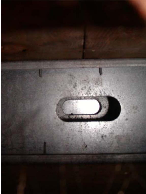
**Figure E.38: Enclosed floor joist punch-out**
