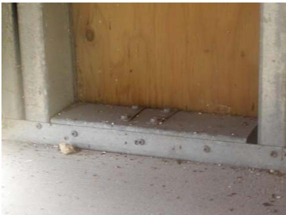
**Figure D.54: SW Cripple Wall base connection**
