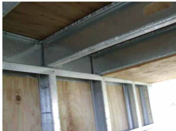
**Figure D.6: Exposed and covered joists**
