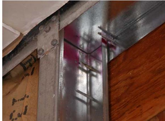
**Figure A.26: East wall – Stud-track connection**
