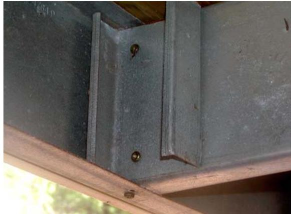
**Figure C.20: Joist stiffener and fasteners**
