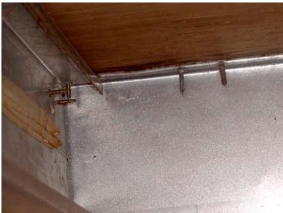
**Figure B.22: Joist to track fasteners**
