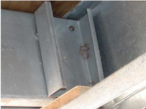
**Figure A.17: Joist stiffener over cripple wall**
