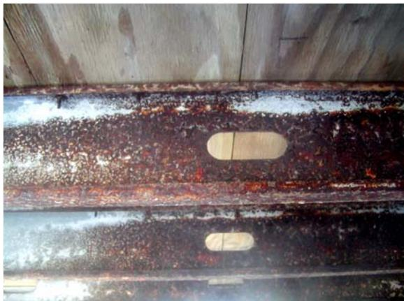
**Figure E.69: Exposed Joists - Midspan**
