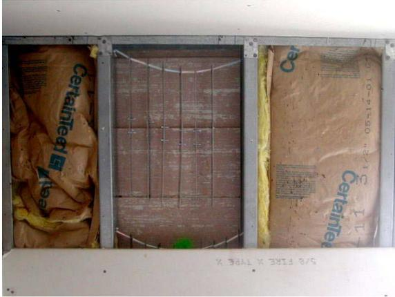
**Figure D.62: Loc. 2 – lap siding w/o vapor barrier**
