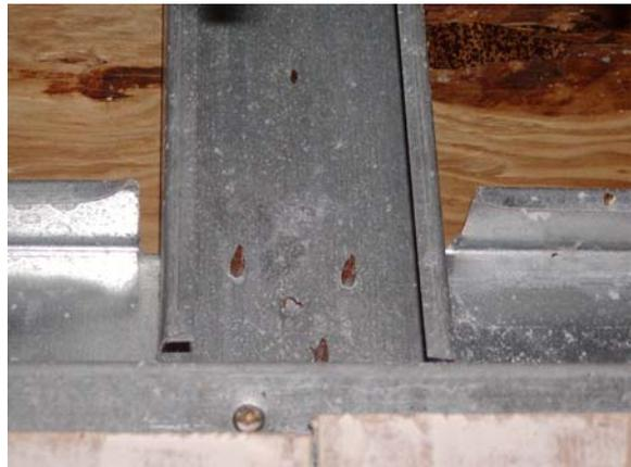
**Figure C.77: Truss bottom connection**
