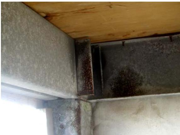
**Figure E.76: Double joist at NW post**
