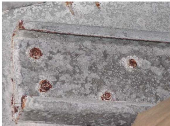
**Figure E.159: Fastener heads at truss connection**
