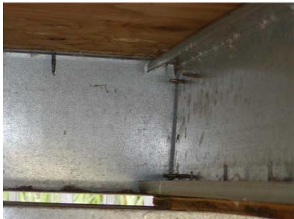
**Figure A.57: Joist connection**
