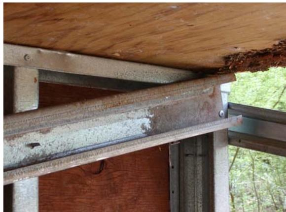
**Figure C.8: Covered joists on cripple wall - SE**
