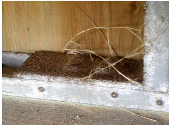
**Figure E.65: Close-up cripple wall tie-down**
