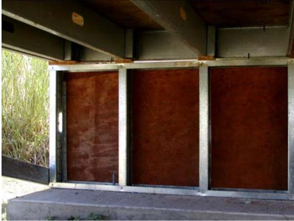
**Figure A.5: Cripple Wall – NE end**
