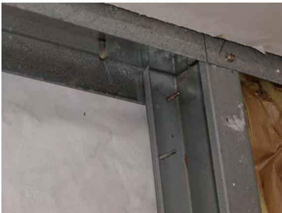
**Figure D.46: N wall – Stud to top track connection**
