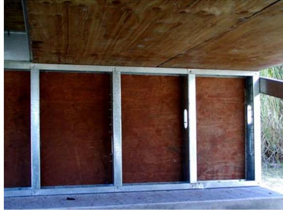
**Figure A.6: Cripple Wall – SE end**
