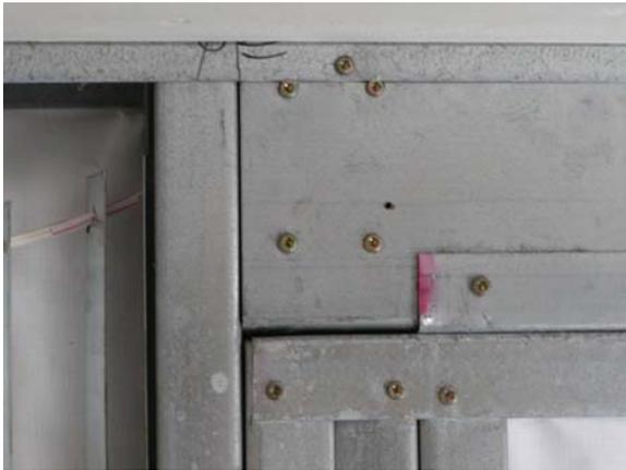
**Figure D.116: Location 3 – Header connection**
