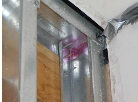
**Figure A.59: Location 1 – Top track connections**
