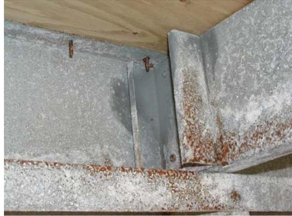
**Figure E.33: Joist stiffener at cripple wall**
