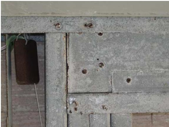
**Figure E.144: W wall header connection - left**
