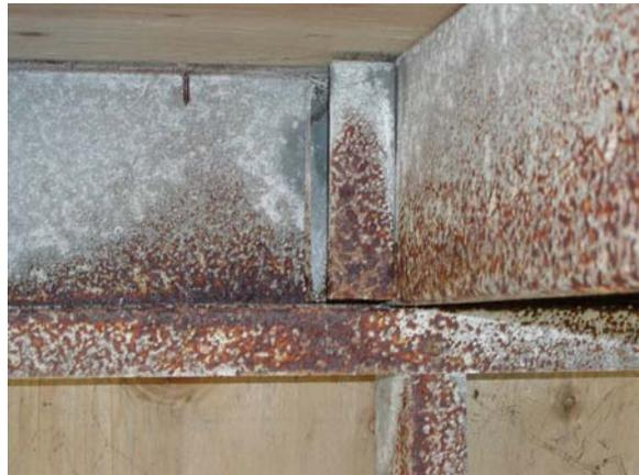
**Figure E.139: Joist stiffener at cripple wall**
