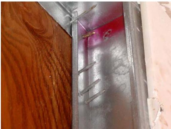
**Figure B.28: East Wall – Stud to track detail**
