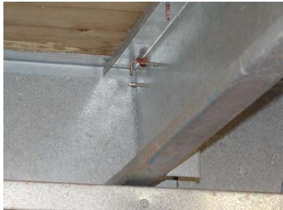
**Figure C.67: Exposed joist connection**
