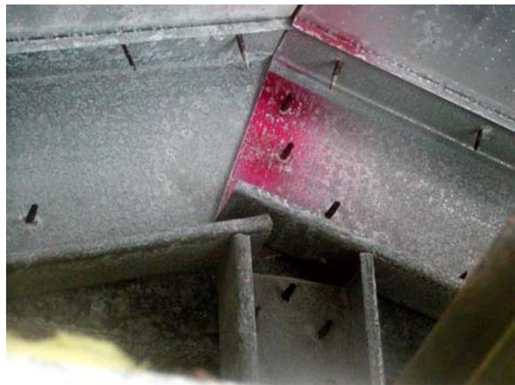
**Figure E.104: Ridge connection fasteners**
