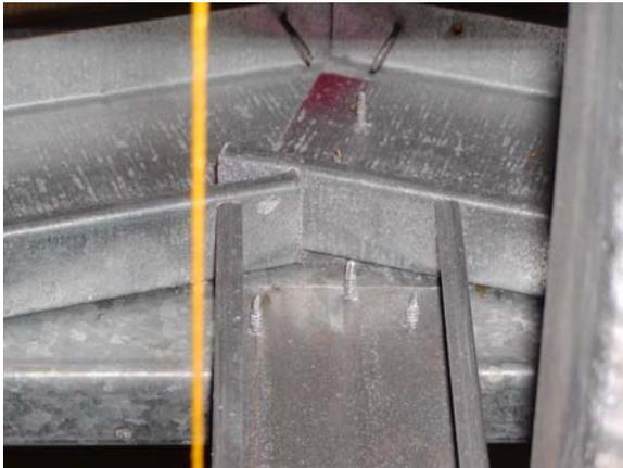
**Figure C.74: Location 2 – Ridge truss connection**
