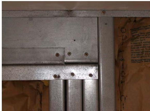
**Figure D.105: Location 1 header connection**
