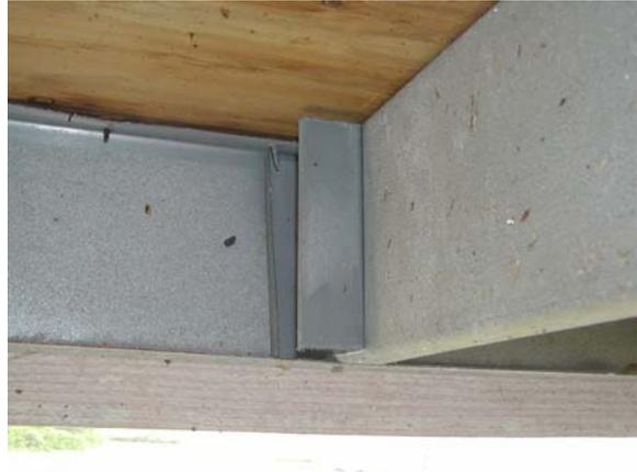
**Figure D.93: Joist end stiffener- open crawl**
