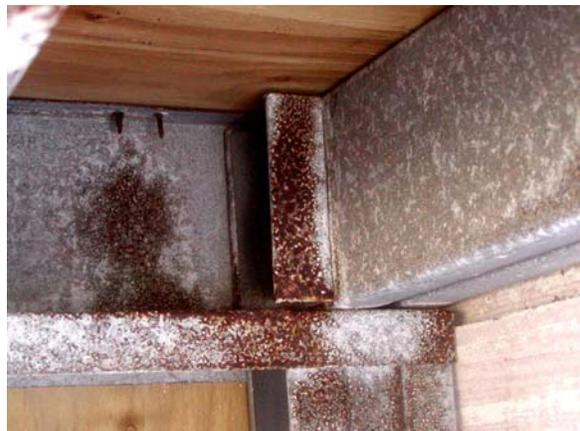
**Figure E.75: Double joist at cripple wall post**
