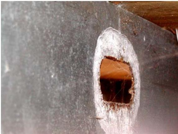
**Figure E.82: Corrosion around opening in joist**
