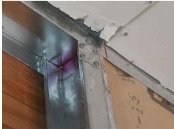
**Figure C.26: East Wall – Stud-track connection**
