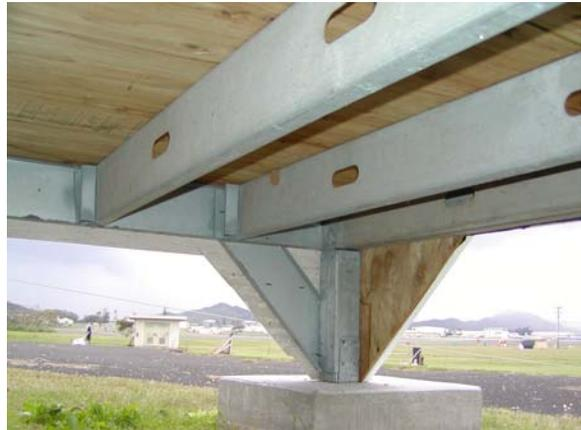
**Figure D.30: SE exposed joists**
