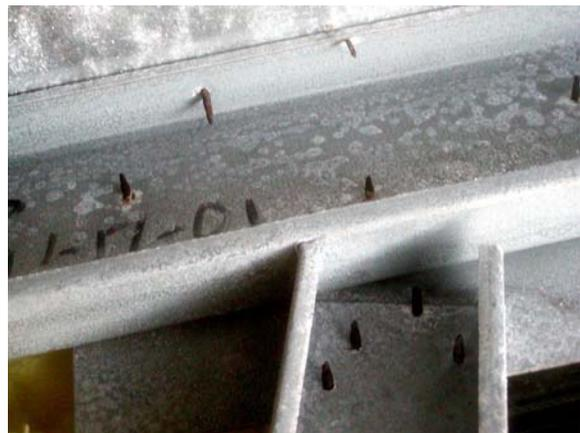
**Figure E.106: Eave connection fastener threads**
