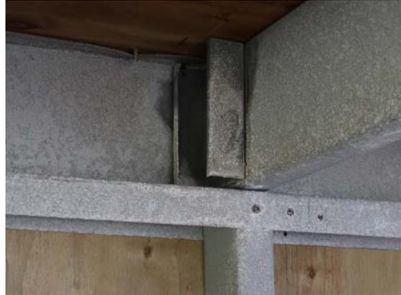
**Figure E.14: Exposed Floor Joist Stiffener**
