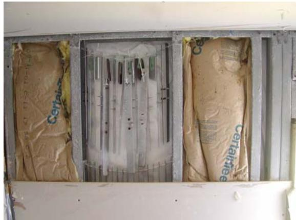
**Figure E.151: N wall – vapor barrier & insulation**
