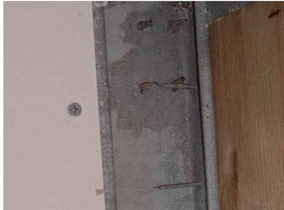
**Figure E.49: E wall – Sheathing & stud fasteners**
