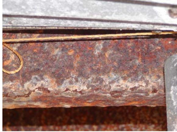
**Figure E.137: Exposed Floor Joists – Close-up**
