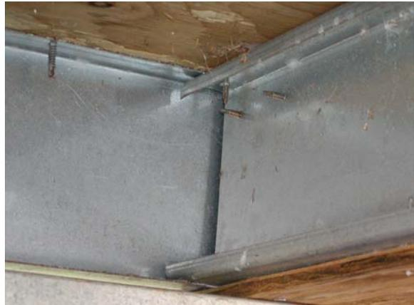
**Figure A.18: Joist connection over cripple wall**
