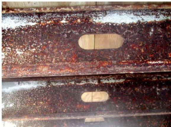
**Figure E.71: Exposed Joists – Midspan corrosion**
