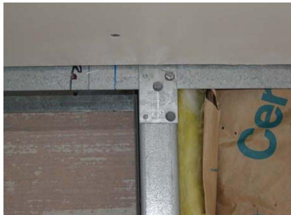
**Figure D.36: E wall – Load path tie-down**
