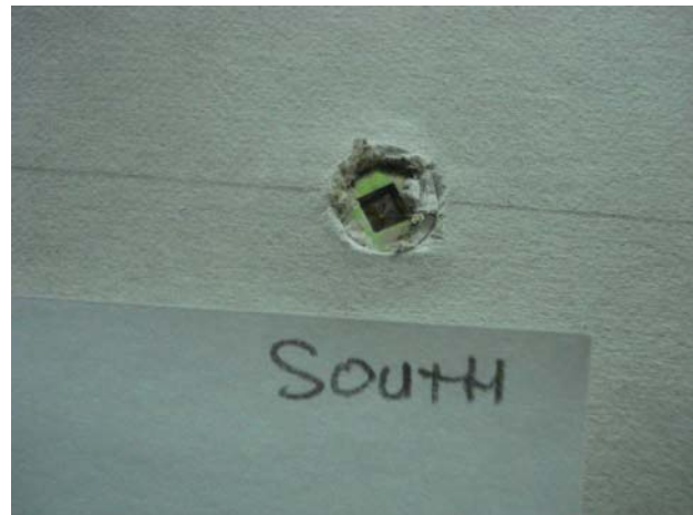
example of overdriven screw (in gypsum board)
