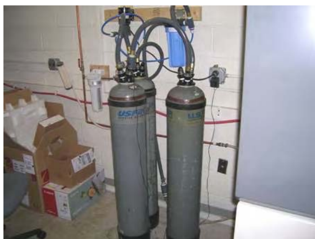
Photo 13 – De-Ionized Water for Spraying
