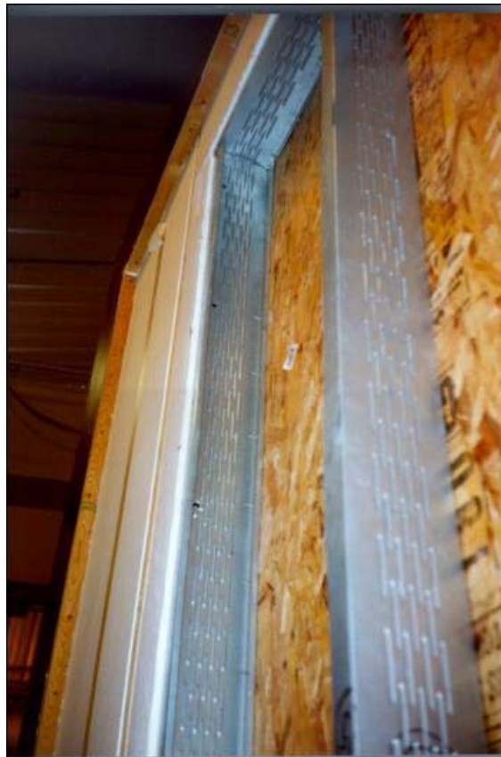
Figure 14 – Slit-Web Stud Wall Assembly
