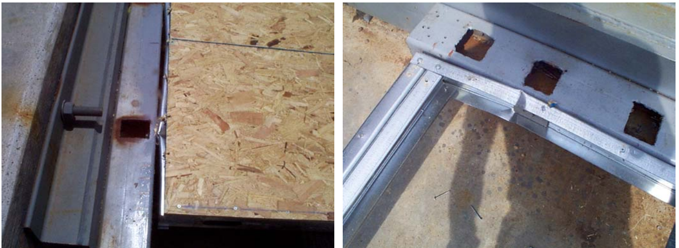
Figure 24 -Damage caused to tracks due to absence of tie-down anchors on end studs
