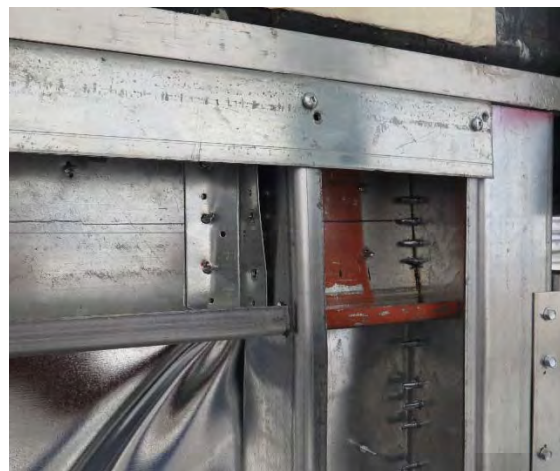
Figure 3.13: Chord stud flange damage at corners. A) Before installing stiffeners. B) After installing stiffeners.
