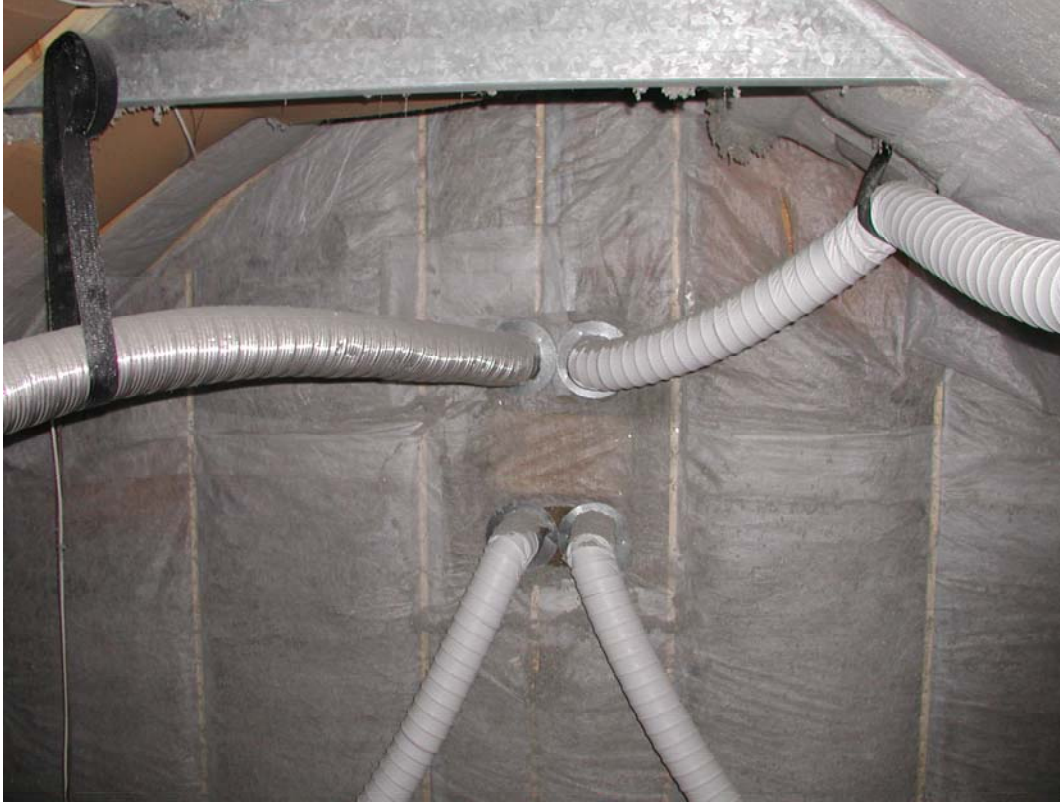
Figure D3. Conditioned Attic with Ventilation
