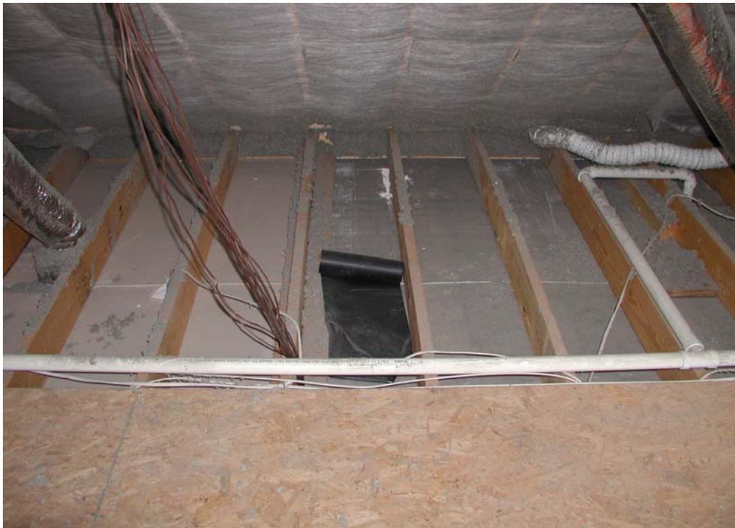
Figure D3. Wood Framed House Insulated Attic Rafters and Uninsulated Floor
