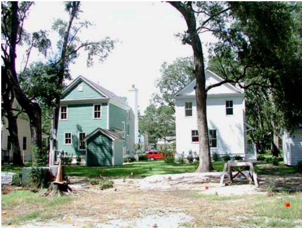
Figure D5. Back of Subject Houses (steel right, wood left)
