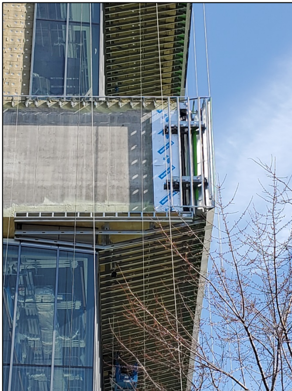
Figure 4 - Cold-formed Steel Framing
