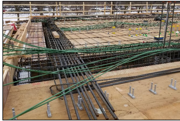
Figure 3 - Post-tensioned Concrete Formwork showing Halfen Embedment Rail System
