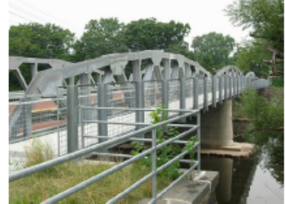
Bergen County Bridge - Fairlawn/Patterson, NJ
